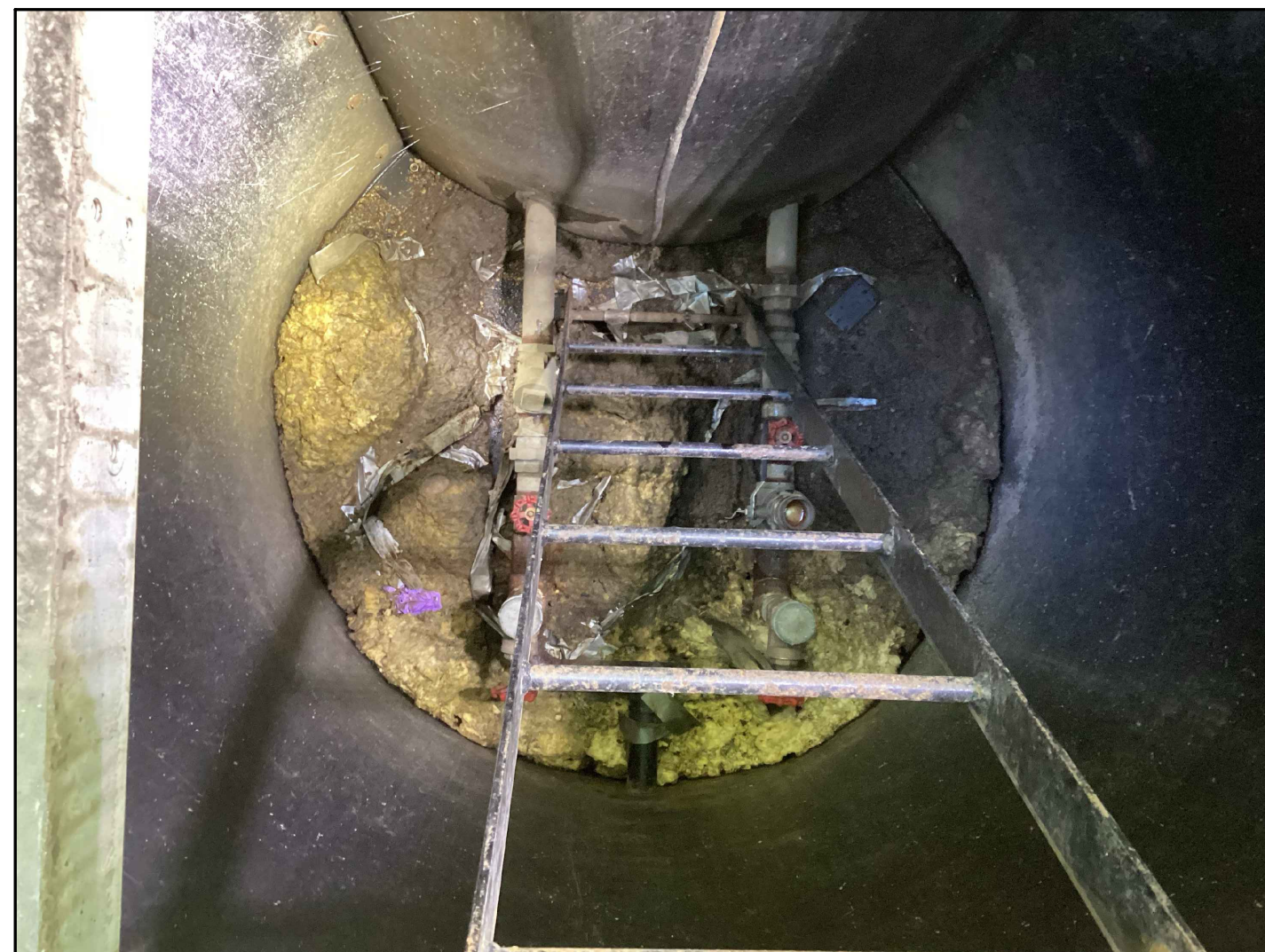
VALVE VAULT TOPSIDE FACING NORTH
