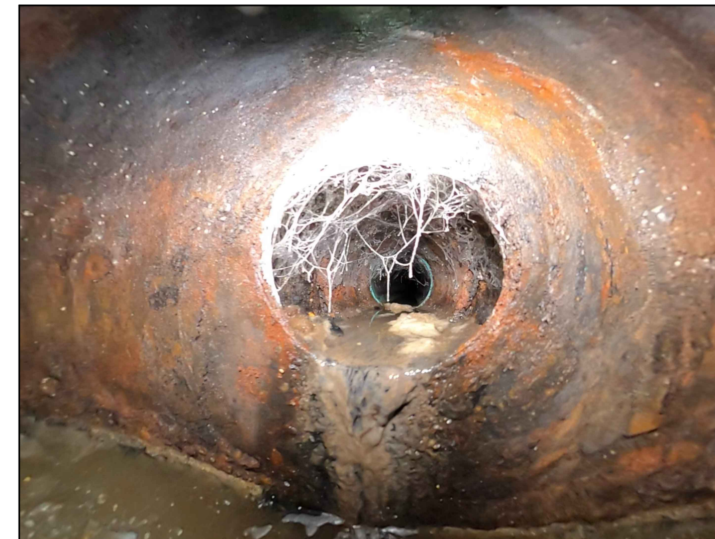
NORTHWEST MAINLINE IN-PIPE
