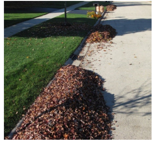
Improper leaf piles, in the street. Leaves in the street clog drains, causing flooding.
