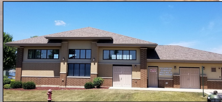
The Village currently uses water pumped from wells to serve residents. However, the aquifer is quickly becoming depleted. The decision was made to connect to Lake Michigan water.
