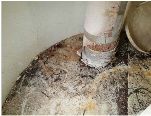
Top Platform Floor and Riser Penetration
