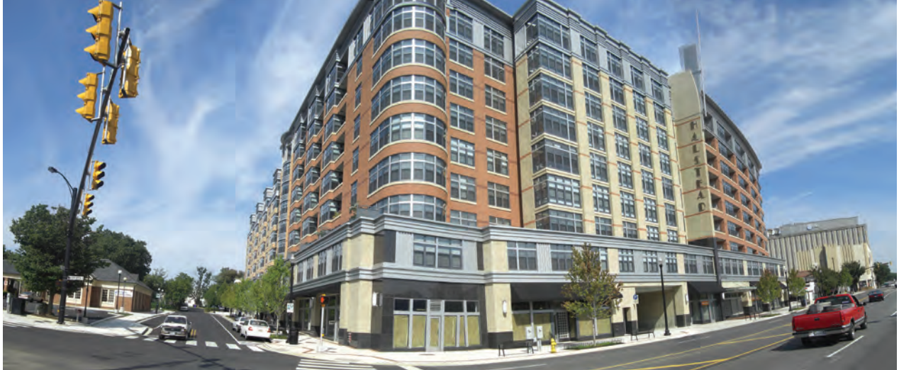
Figure 2.17. The Halstead was the first project developed under the Columbia Pike form-based code.
