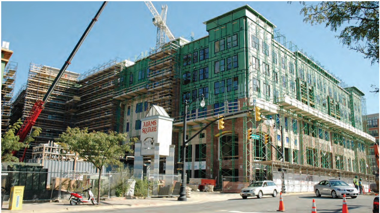
Figure 2.18. Construction of the Penrose Square site
