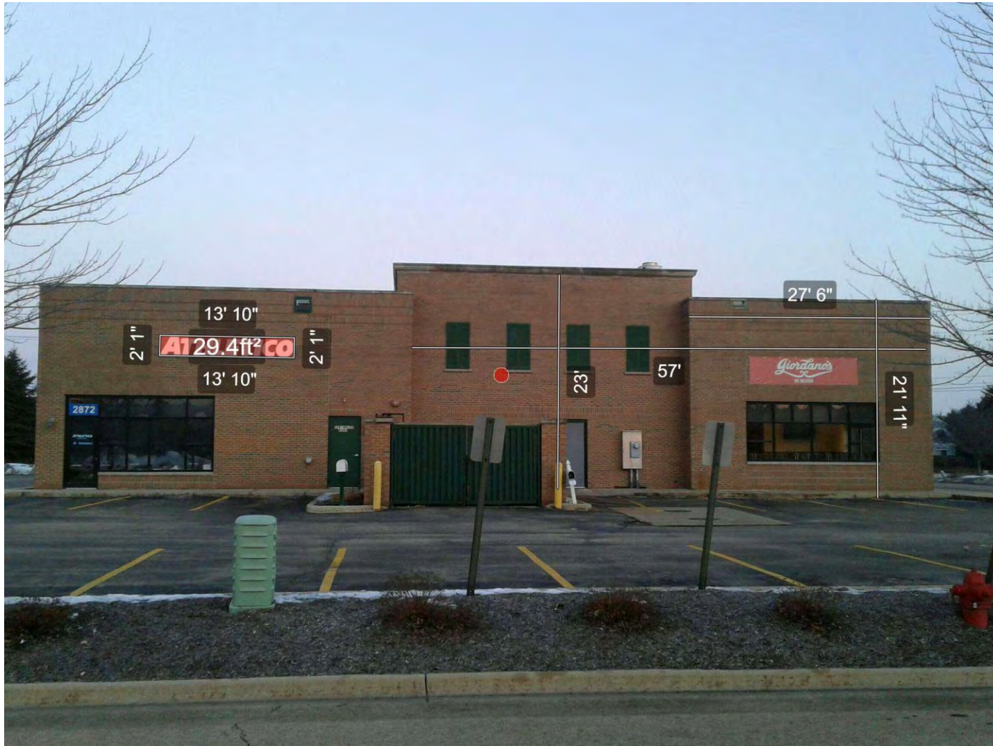
Survey of existing conditions – Rear elevation
