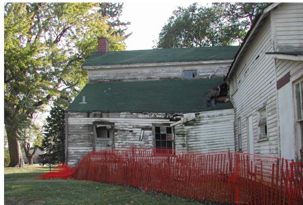
REHABILITATION AND RESTORATION WORK ON THE STRAWBRIDGE-SHEPHERD HOUSE HAS TRANSFORMED THE BUILDING INTO A MUSEUM AND EVENT SPACE (PHOTO CREDIT ELLJAH ILES HOUSE FOUNDATION)
