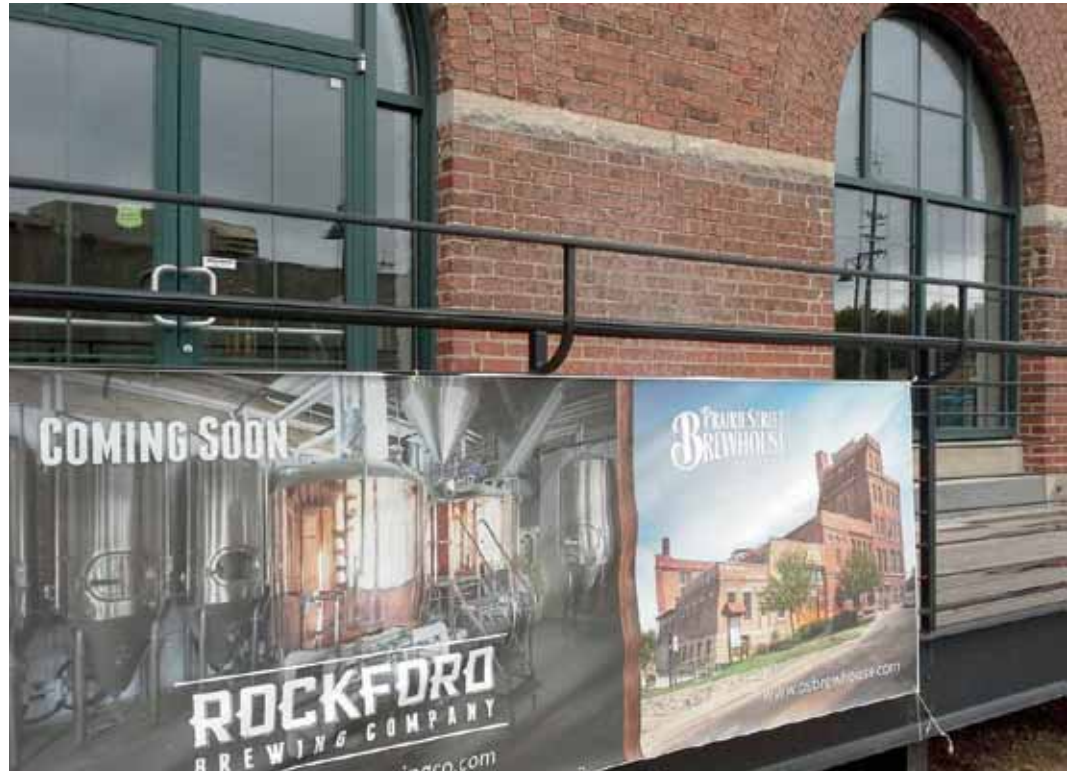
Rockford: Peacock Brewery rehabilitation
