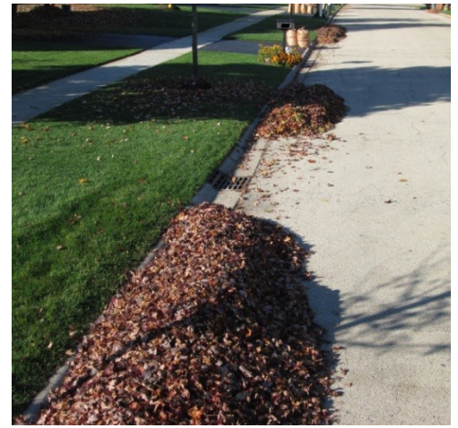
Improper leaf piles, in the street. Leaves in the street clog drains, causing flooding.
