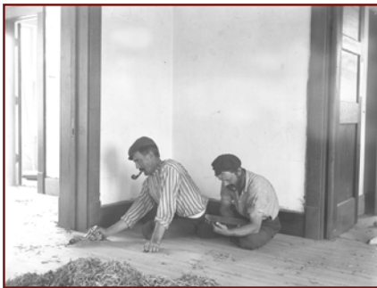
Carpenters Lou Inman and Lou C. Young planing the wooden floors in the Cutters' new house, 1903 – photographed by Irvin Haines (courtesy of the Little White School Museum)
