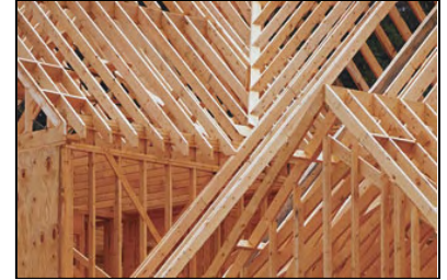
Use recycled building materials wherever feasible
