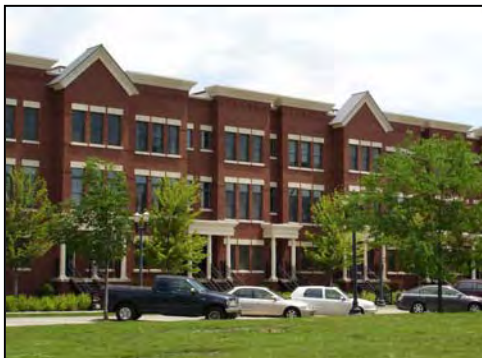
Typical Multi-Family Residential Character
