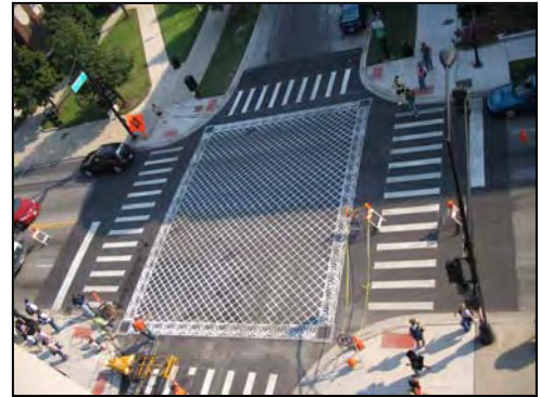
Cross-walk enhancement with intersection application for visibility
