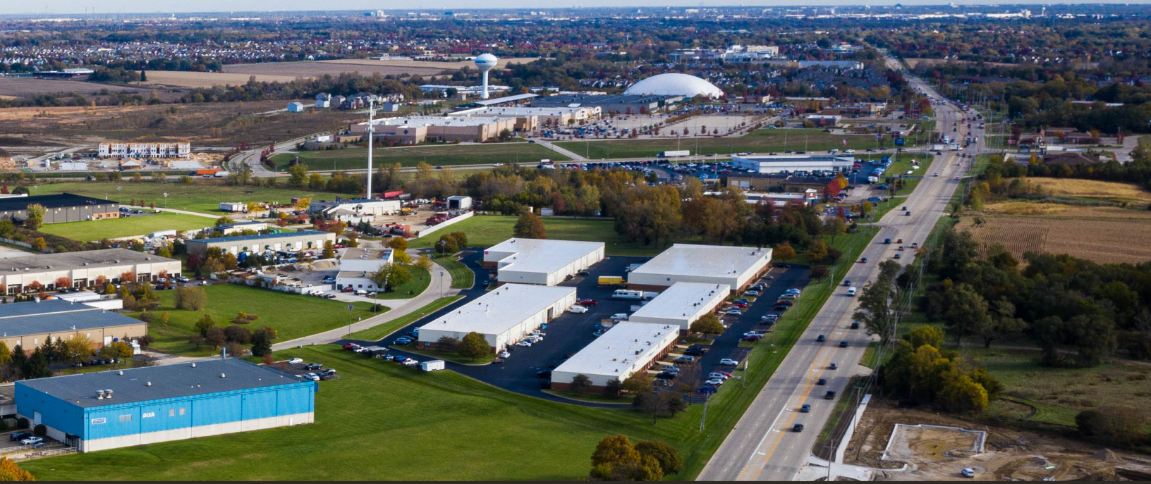
Development continues along several corridors in Oswego. Above, a flagship location for Delta Sonic will open along the Route 34 corridor, bringing state-of-the-art car care services to town, just across the street from one of Oswego's four business parks.
