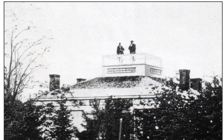
The stone house at 56 Jackson Street in 2014 (top) and in 1860 (bottom). Historic photo courtesy of the Little White School House Museum.
