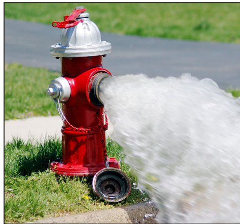
Water main flushing flushes iron deposits and helps pull fresh water all the way through the line.
